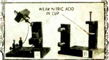
Electrolytic Detectors about 1902-'03 (N.E.S.W.G.C.)
